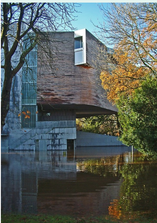
Glucksman Gallery during flooding, 2009. © Dr David J. Otway (2009)
