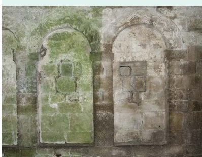
Trial UV treatment of algal growth (Office of Public Works)
